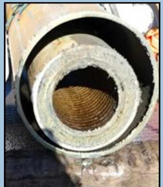
Cut Completed on 20" J-Tube & 10" Riser
